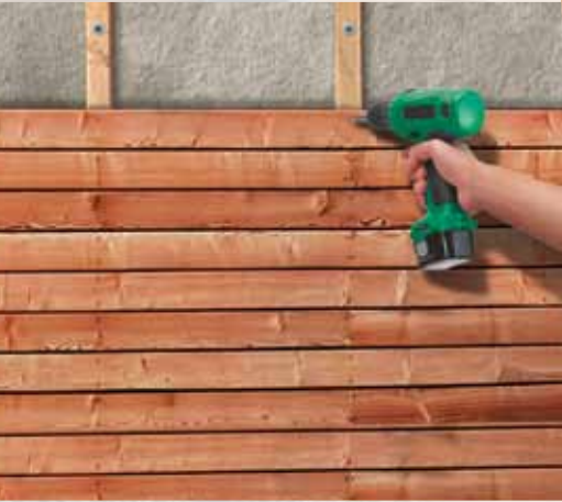
Assembly of the facade cladding
