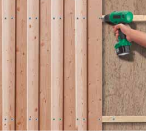
Assembly of the facade cladding
