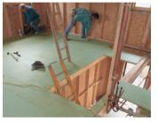
**OSB (Oriented Strand Board)**: a low cost, dimensionally stable resin-bonded sheet made of small strands of wood. Suitable for structural floors, roofs, hoardings etc.
